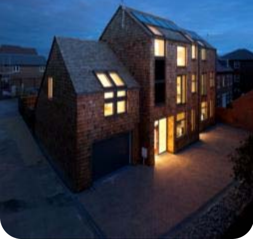
Carbonlight Homes, UK
